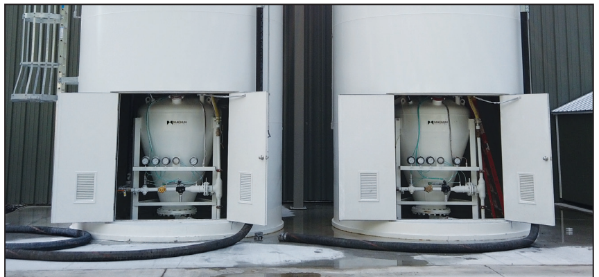
Dense phase transmitters in the silo skirts supply the minerals through the total system solution at The Quartz Corporation.
