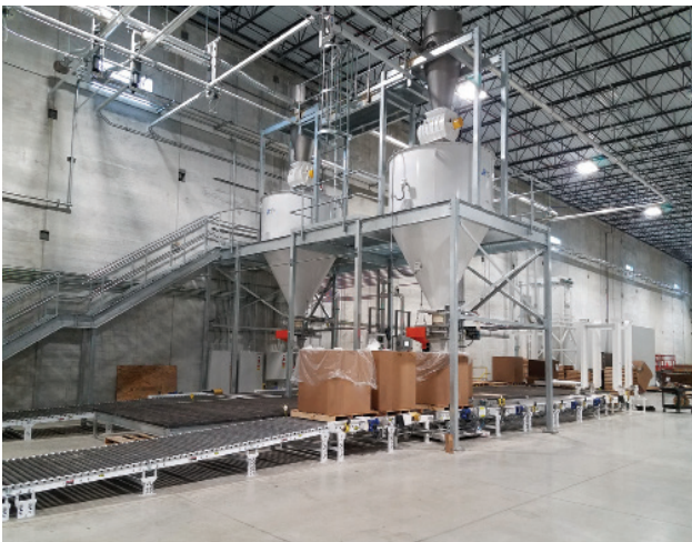
Figure 1. Dilute phase transfer system allows for material to be transferred to one of two surge bins. The surge bins gravity discharge 1000 lb of material into a Gaylord tote filler. Roller and chain conveyors index the Gaylord totes into and away from the filling station.
