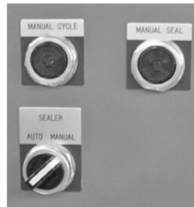
Figure 25 – Sealer Buttons On Control Panel
