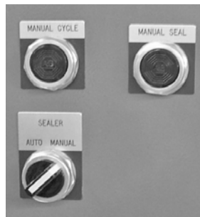
Figure 29 – Sealer Buttons On Control Panel
