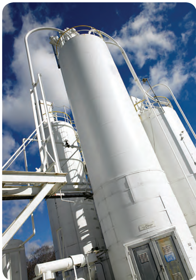
Pneumatic transfer system
