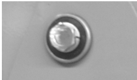
Figure 7-7. Shut Off Gate Mounting Screw Ground Off Smooth
